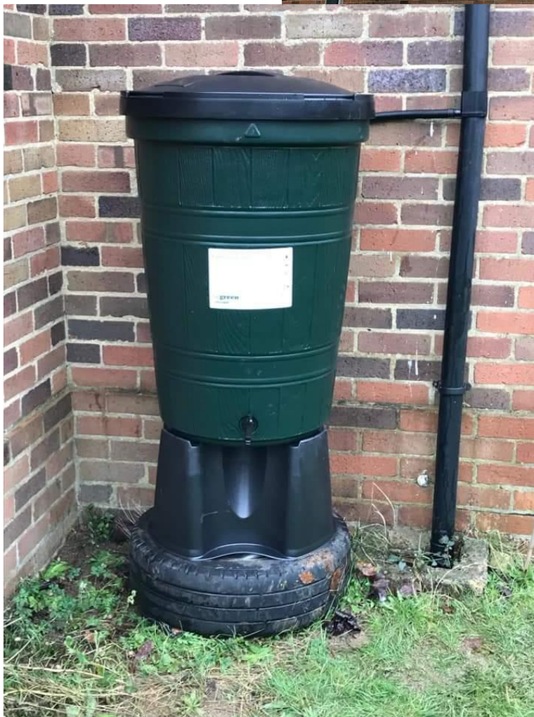
Water butt – we used a dumped old tyre as a base
